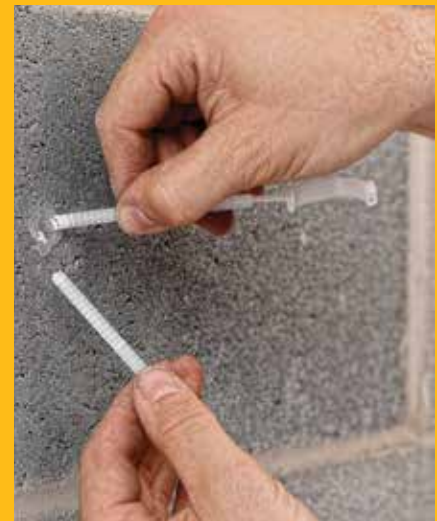
STRAP-TOGGLE INSTALLATION
